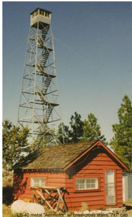
LS-40 Metal Aermotor: Criss-Cross Stairs, 7'x7' Cab
